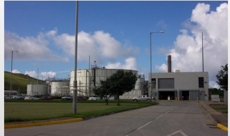
Leachate Treatment: Another Challenge
